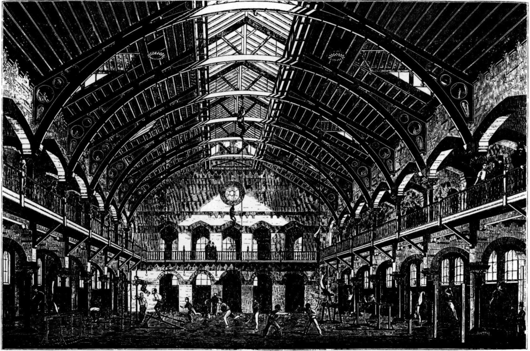
Fig. 11 The German Gymnasium, Cheney Road, King's Cross, London, illustrated in The Builder , 19th May 1866
