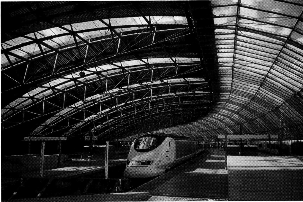
Fig.8 Waterloo International Station, London
